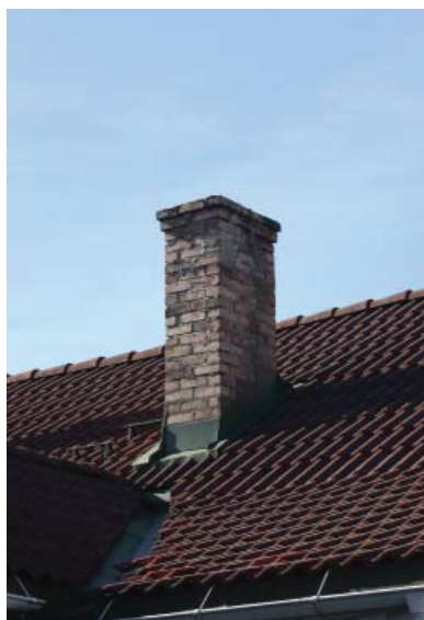
Ubehandlete piper i teglstein
